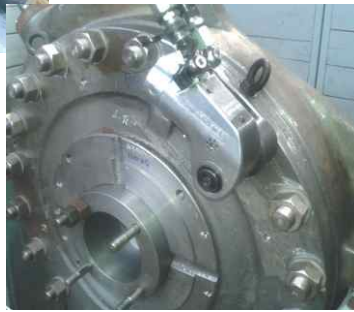
◀ PSD-3 Bolt tightening of Centrifugal pump casing
